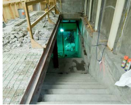
R Platform Level Stairs East
