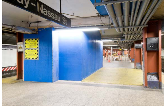
Platform Level – Conduit Installation.
