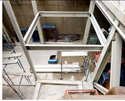
Stairs – Structural Steel Concourse Level .
