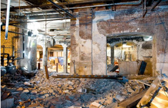
135 William Street Below Grade Demolition
