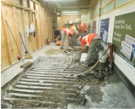
R Northbound Platform Demolition
