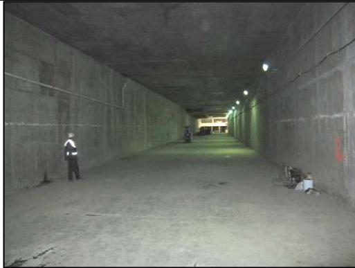
Dey Street Structural Box Completed
