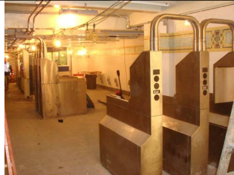
Fare Control Finishes
