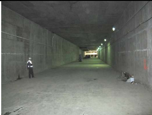
Dey Street Structural Box Completed
