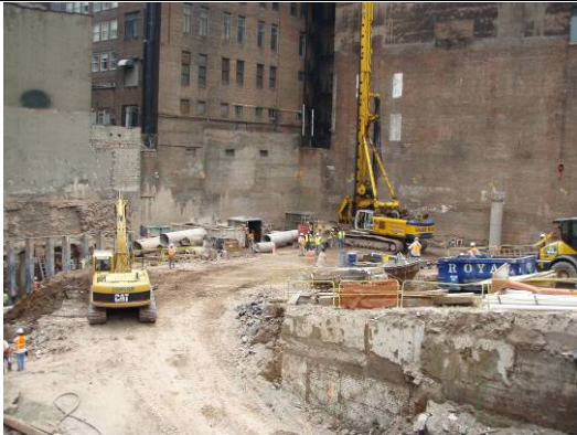
Secant Pile Installation
