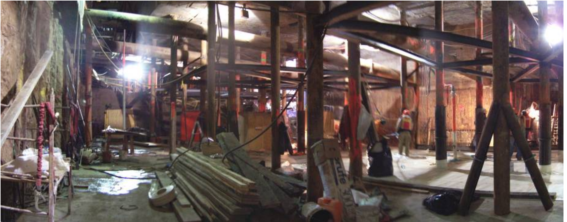
Lexington Avenue line underpass looking south
