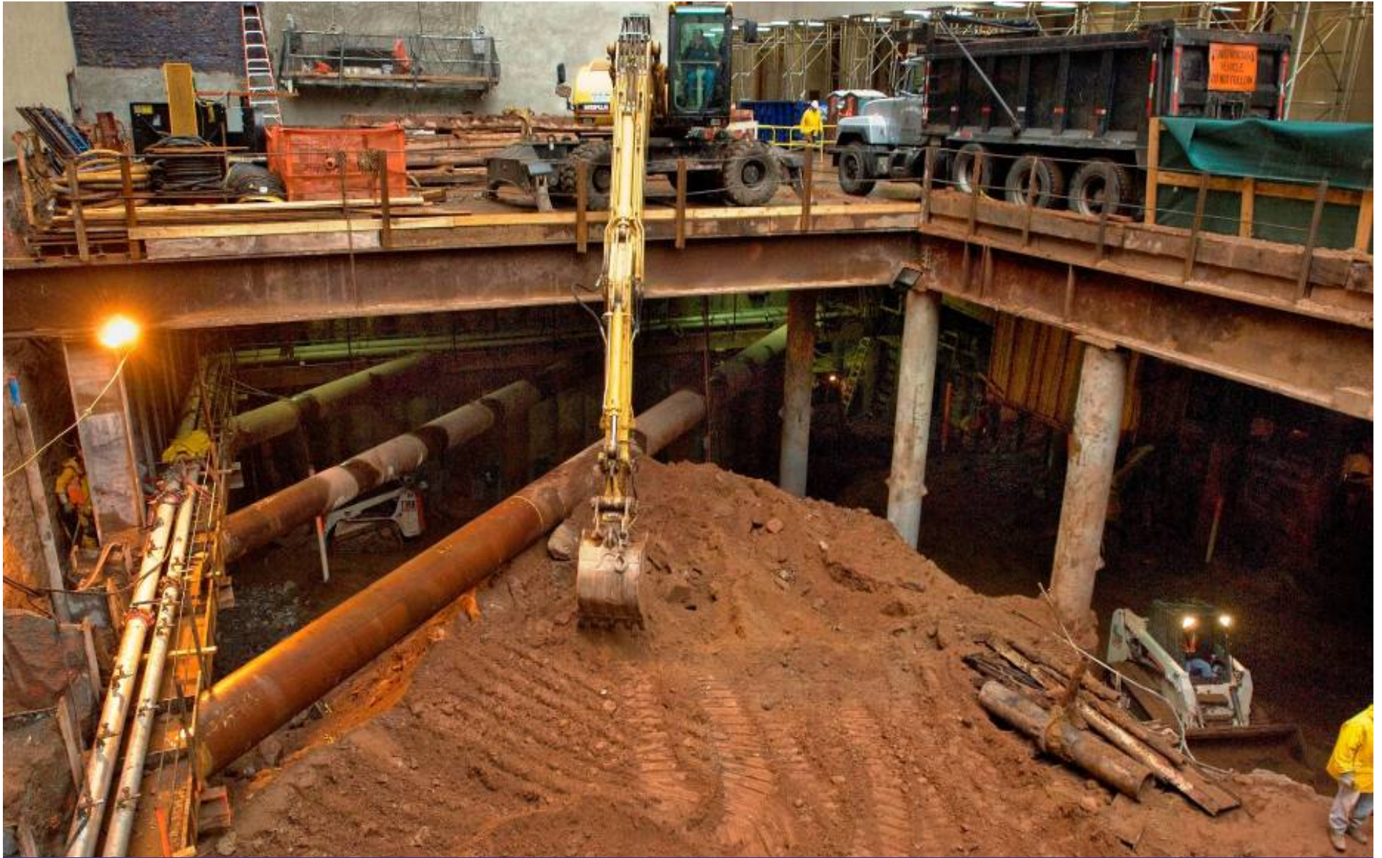
Dey St Passageway and Headhouse entrance looking west
