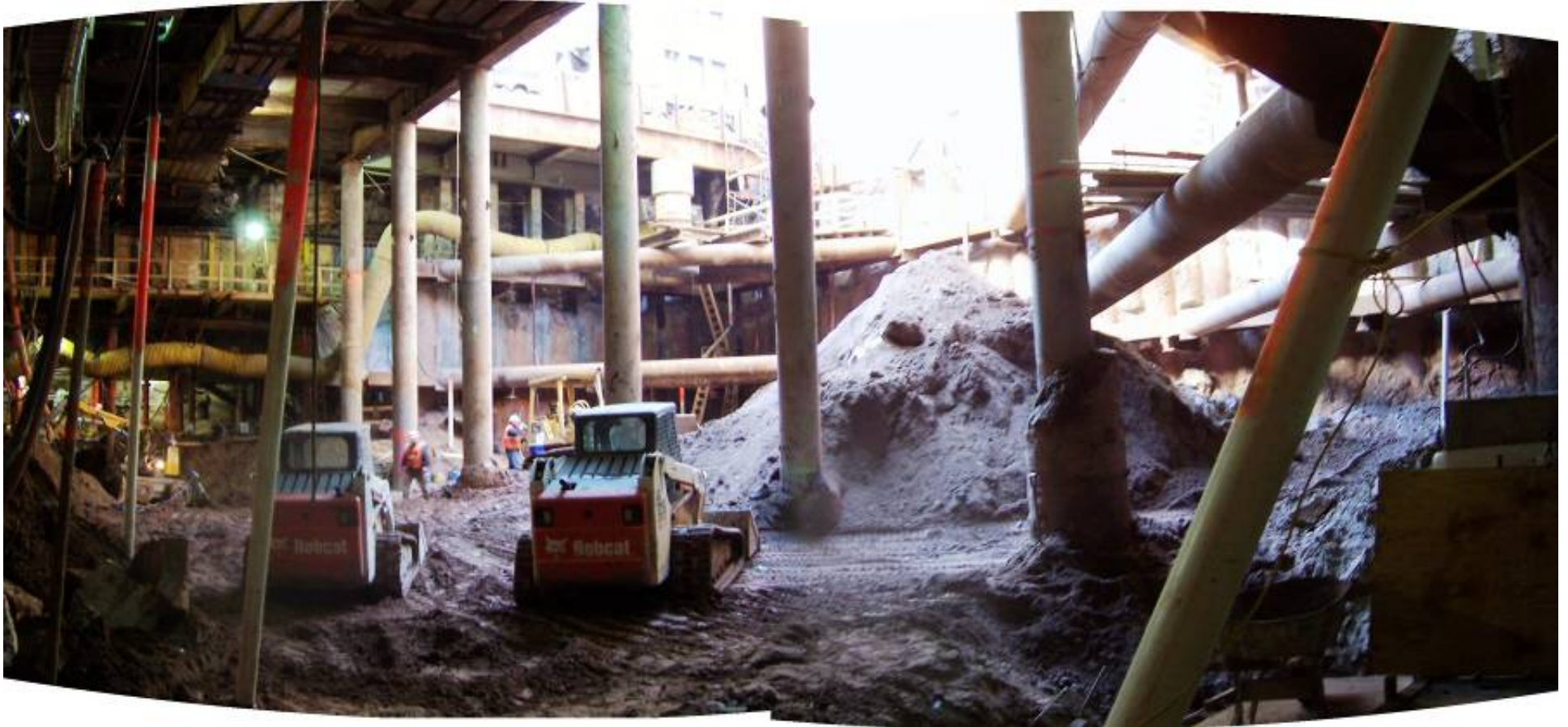
Dey St Passageway and Headhouse entrance looking east
